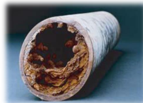
Erosion Corrosion (Microbiologically Induced corrosion)
